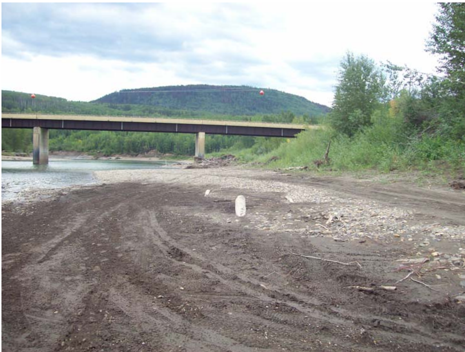
Photo 83. Twidwell Bend South bank shoreline (main access).
