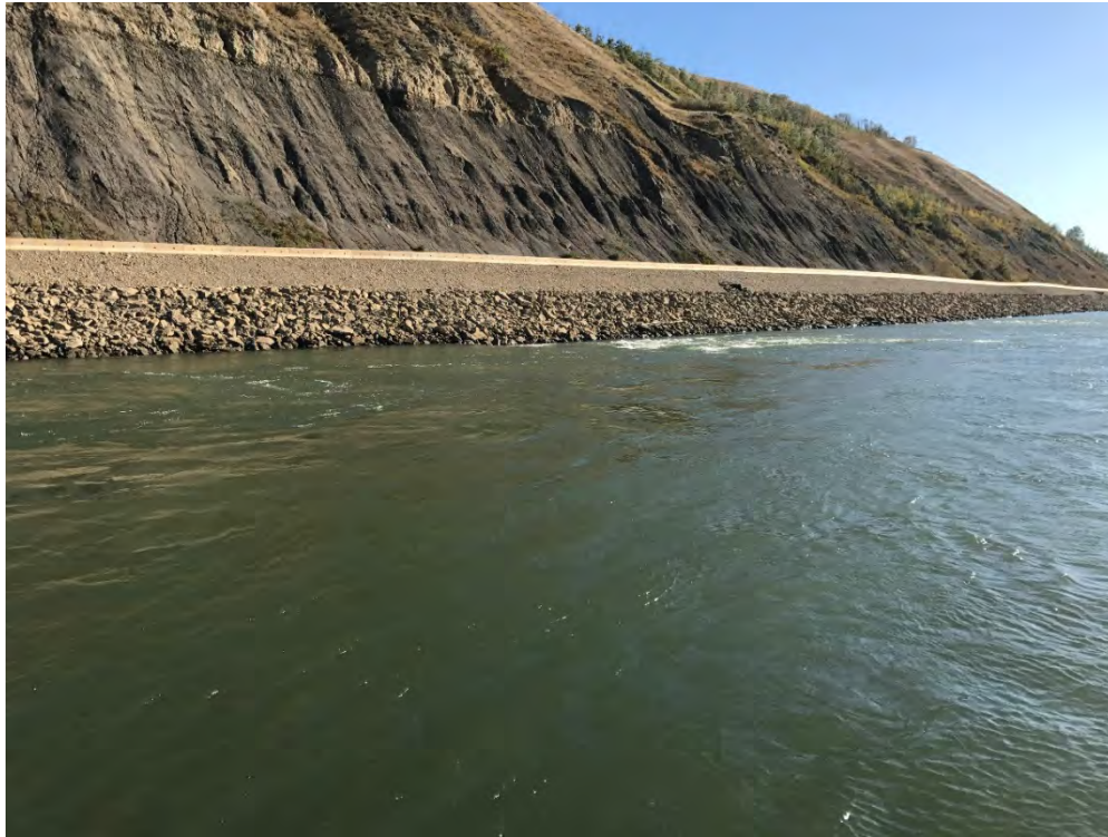
Plate 1 View of non-laminar flow observed around rock spurs located along River Road. Photo taken 10 September 2017 at approximately 9:30 am.
