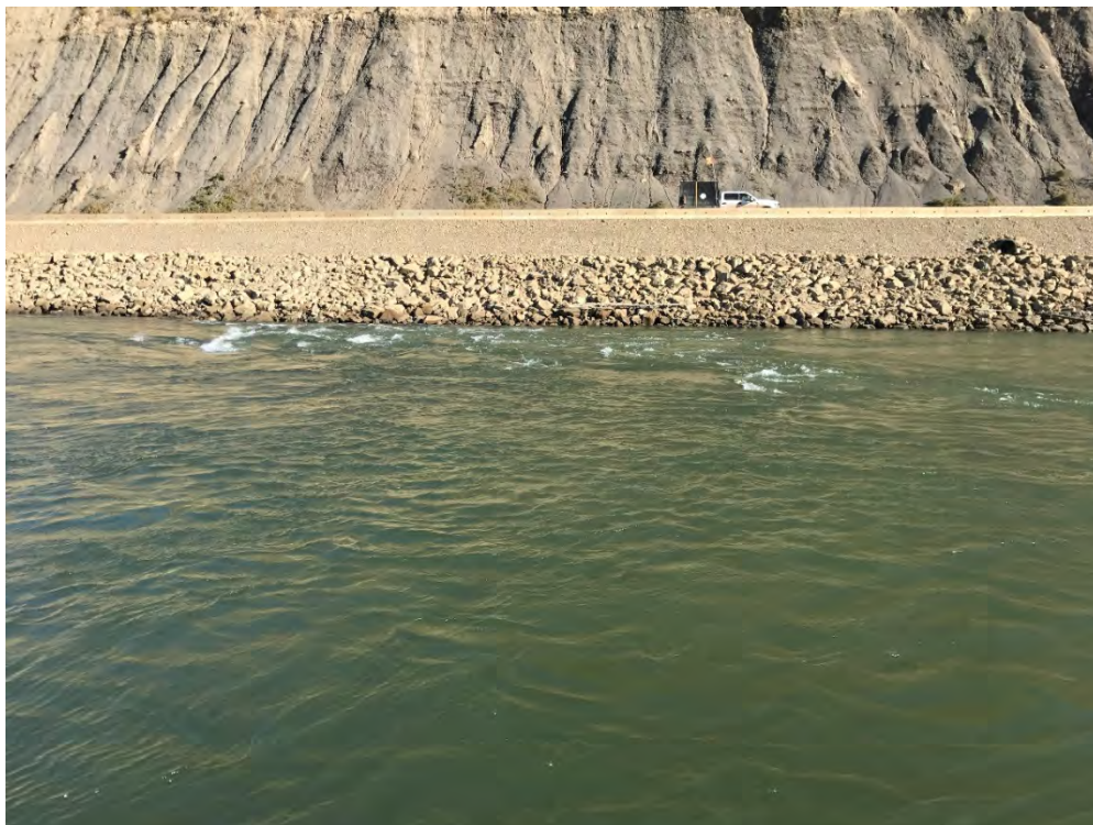
Plate 2 View of non-laminar flow observed around rock spurs located along River Road. Photo taken 10 September 2017 at approximately 9:30 am.
