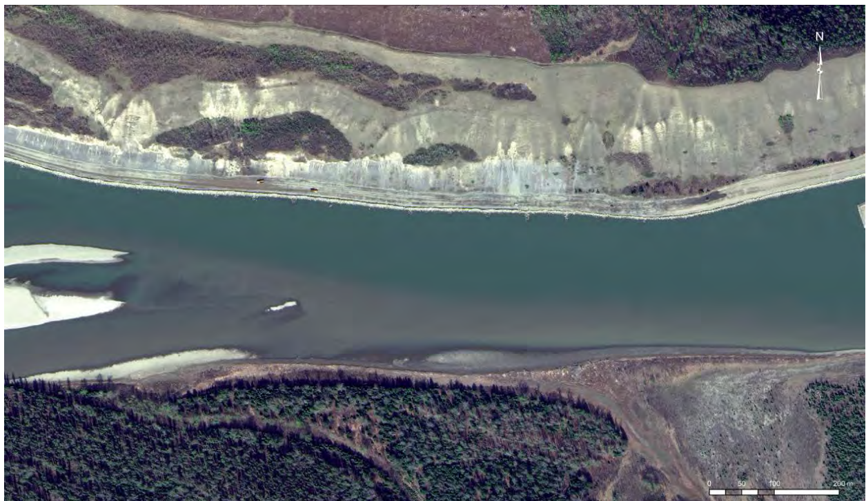
Plate 4 Aerial view of the River Road area after the construction of River Road and rock spurs. Photo taken on 26 April 2016.
