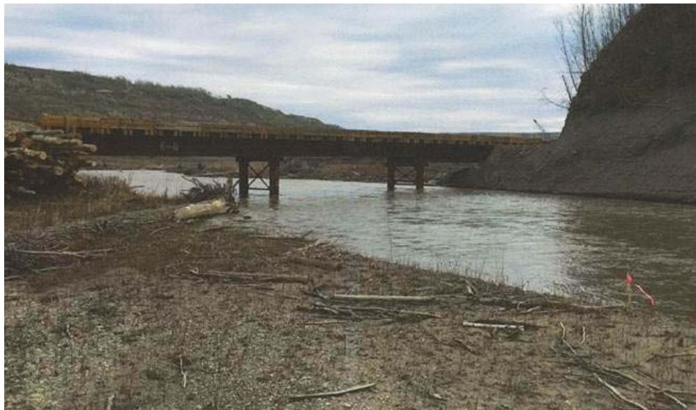
Figure 2. Temporary Moberly River vegetation clearing bridge removed in March 2016.
