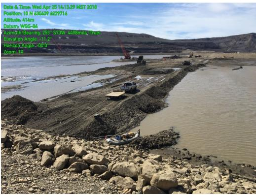
**Figure 2.** Fish were excluded using stop-nets during restoration of the back channel on the south bank island downstream of the dam (November 16, 2018).
