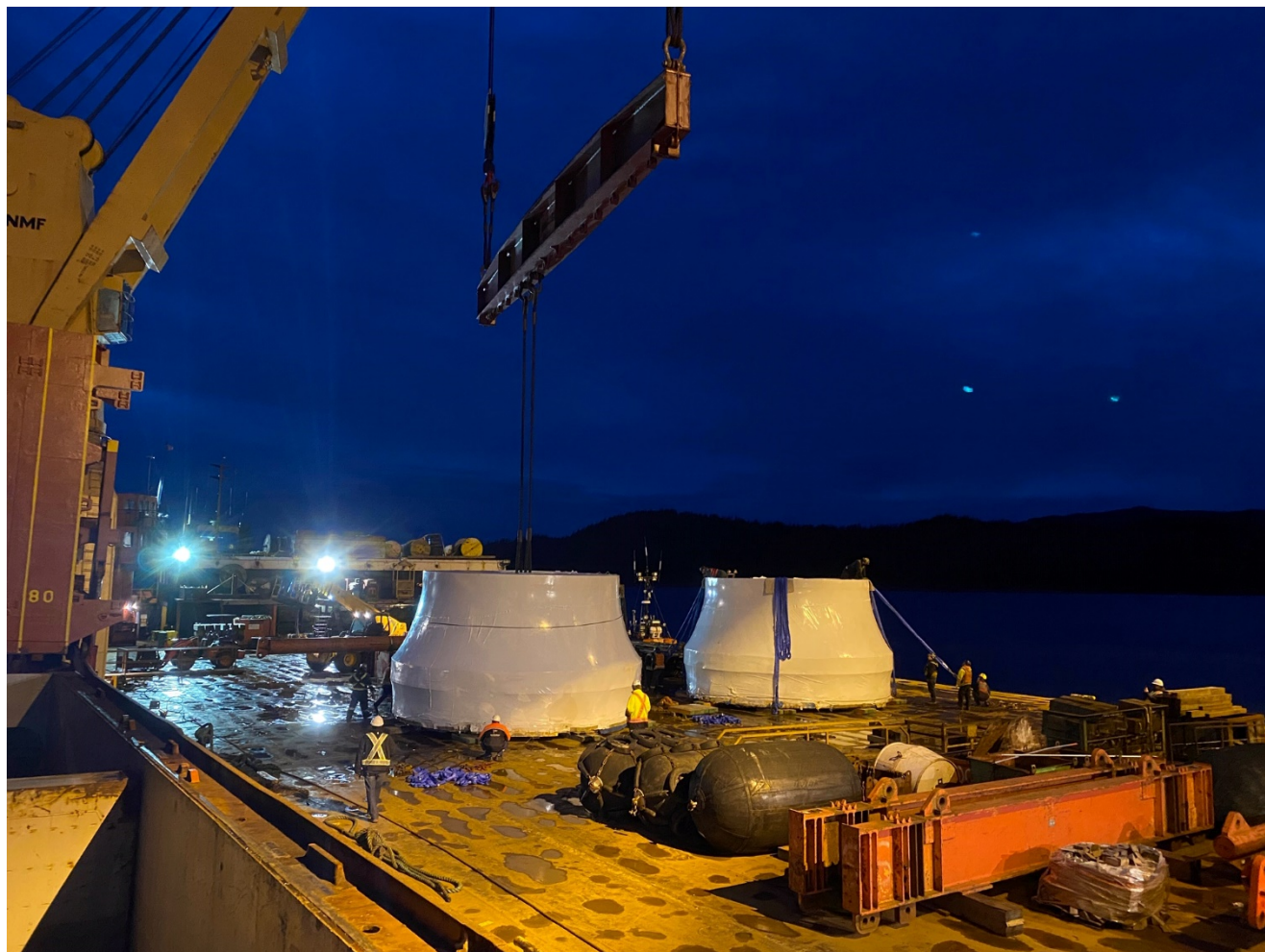
The first turbine runners arrive in Prince Rupert from São Paulo, Brazil. See more project photos in the image gallery .
