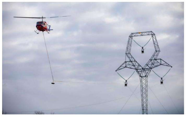
Helicopters are used to string the sockline between the transmission towers. See more project photos in the image gallery.
