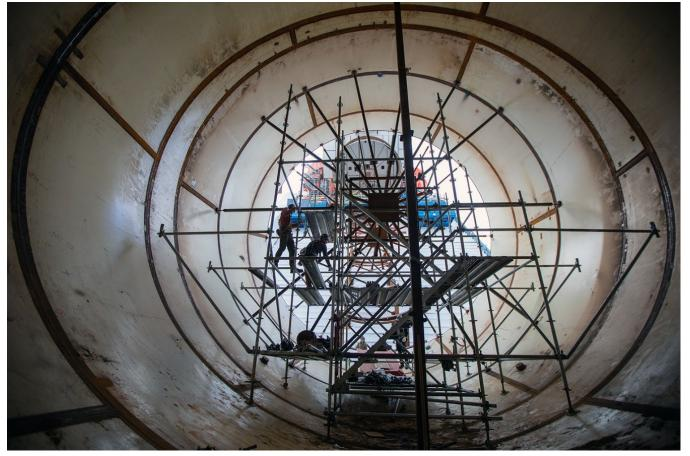
Scaffolding is installed inside a penstock to allow access to the edge of the unit to weld sections together. See more project photos in the <u>image</u> <u>gallery</u>.
