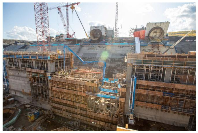
Two of the six penstocks that carry water from the reservoir into the powerhouse are being installed. See more project photos in the image gallery.
