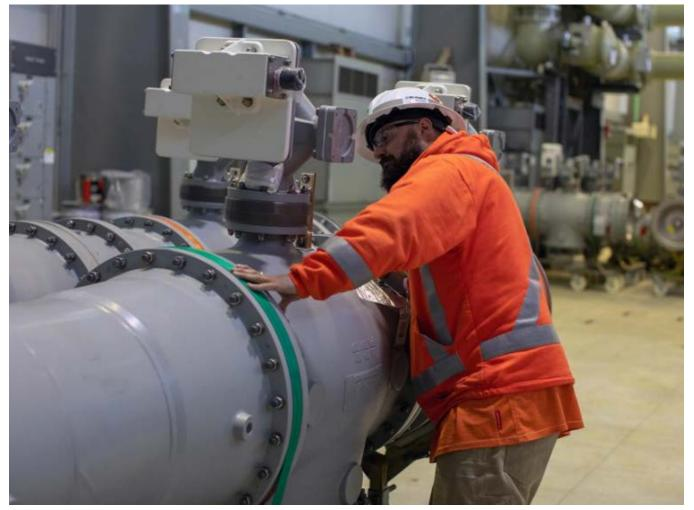
A worker inspects the new gas-insulated switchgear equipment at Peace Canyon substation. This new equipment will be used to connect the two new 500 kV Site C transmission lines to the BC Hydro power system. See more project photos in the <u>image gallery</u>.
