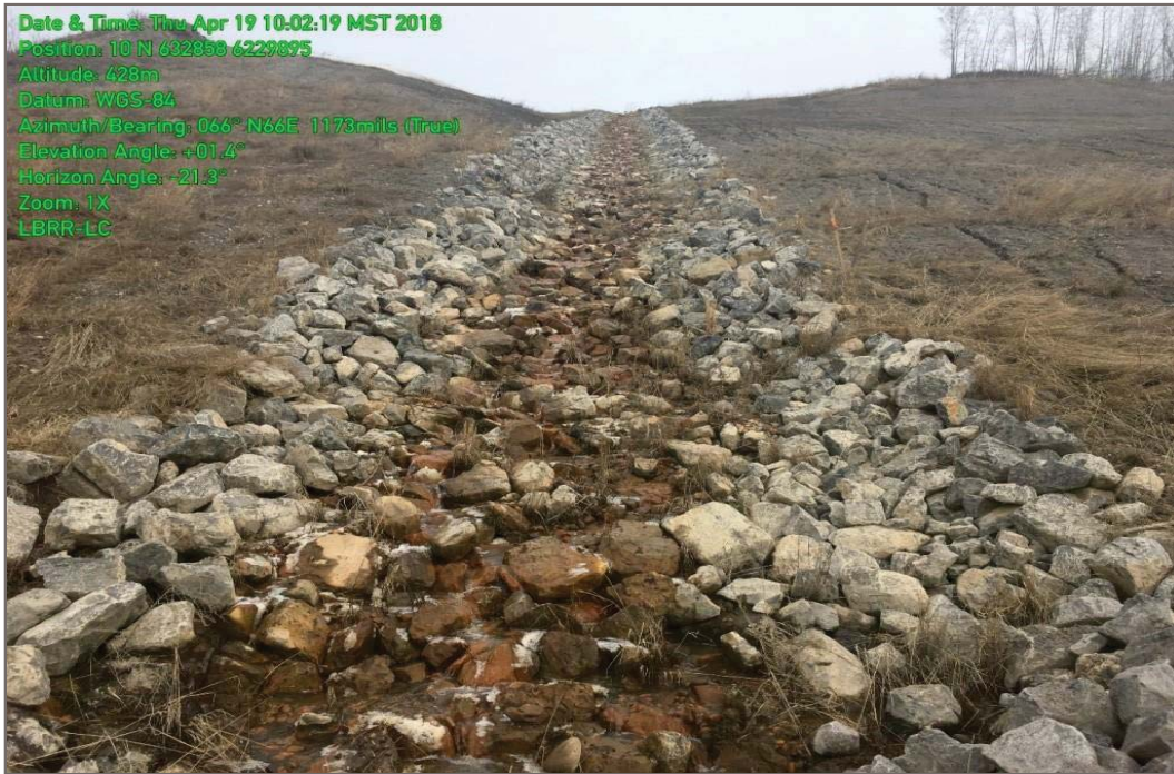
Photo 3: River Road water sample location LBRR-LC, dated April 19, 2018
