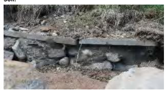
Photo 22: Snake 326 (Lynx Creek) entrance on 11 June 2021 after filling excess gaps.
