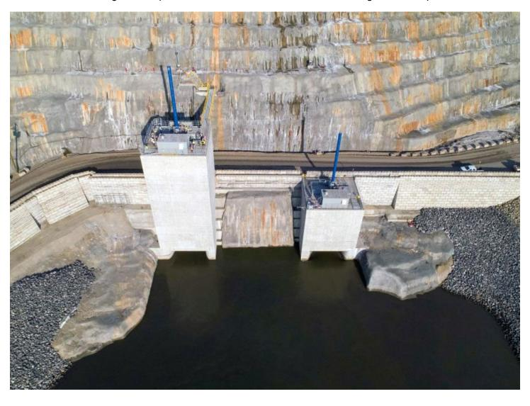
**Photo 5.** Final rip rap is placed on the rockfill berm (center) to close the Peace River on October 3, 2020 (looking downstream).
