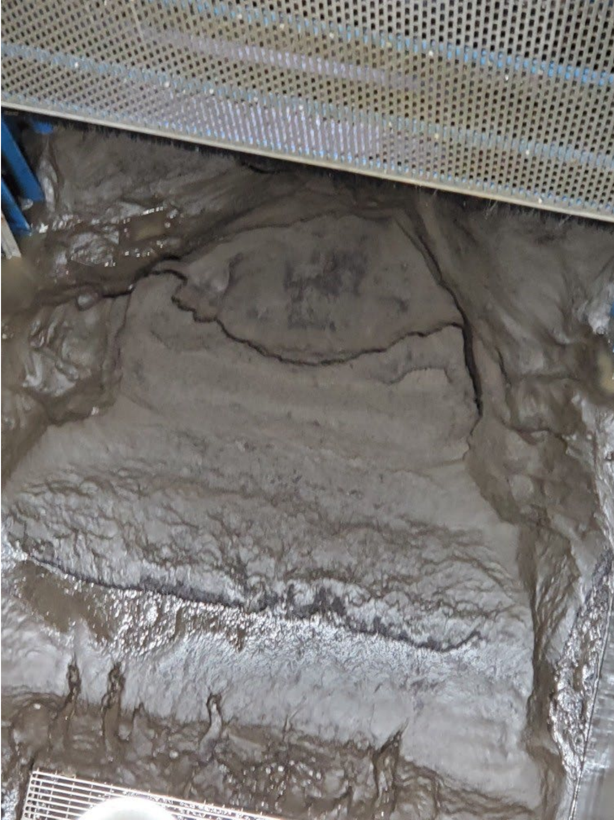
Photo 2. Build up of sediment in the pre-sort holding pool, which required clean out with a hydrovac at the beginning and end of the reporting period (June 29, 2022).
