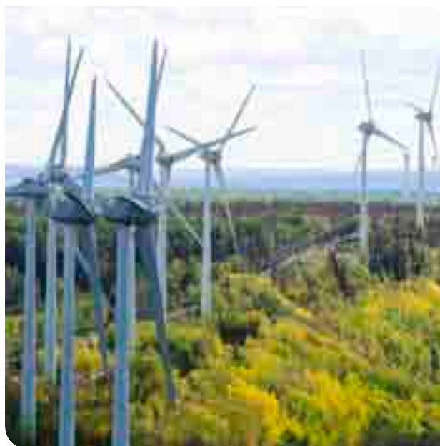
Wind farm near Dawson Creek.
