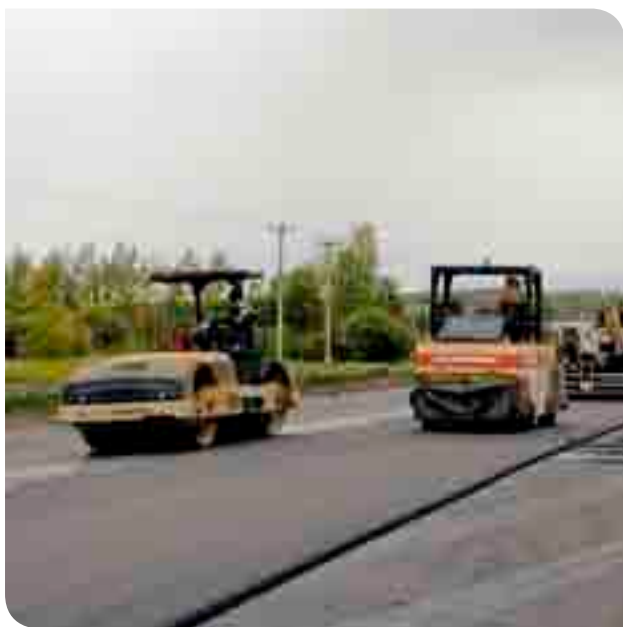
Road improvement project near Fort St. John (September 2009).
