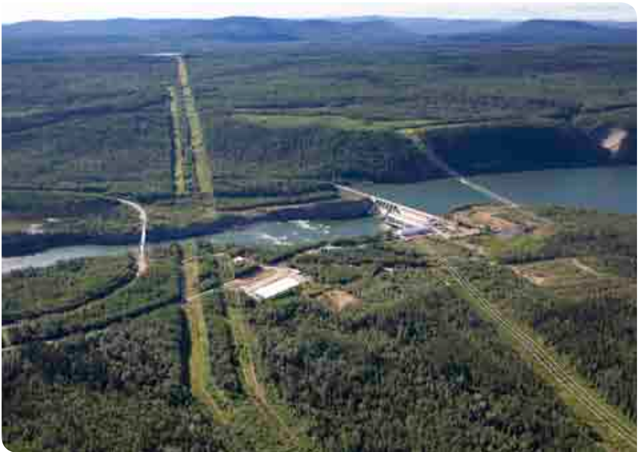
Transmission lines connected to the Peace Canyon Dam (July 2009).
