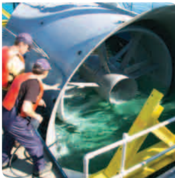
Turbine at Race Rocks Tidal Energy Project (2006).
