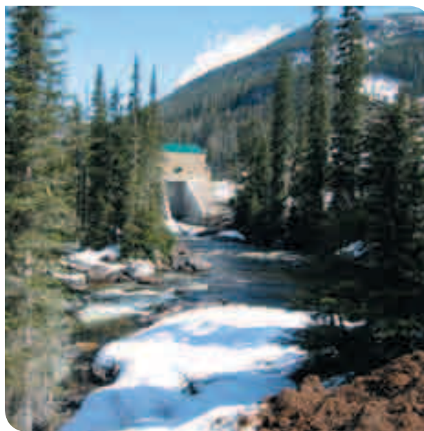
The Pingston run-of-river small hydro plant, south of Revelstoke.
