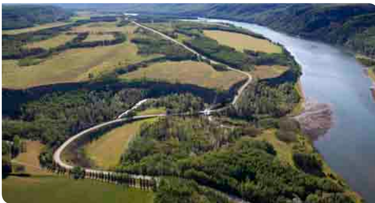
Highway 29 at Farrell Creek.
