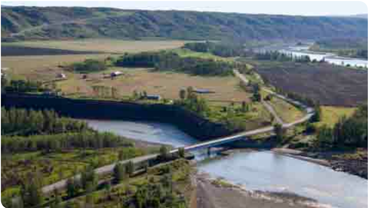
Highway 29 crossing the Halfway River.
