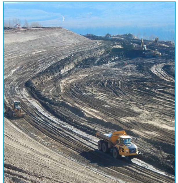
North bank excavation at the Site C dam site.
