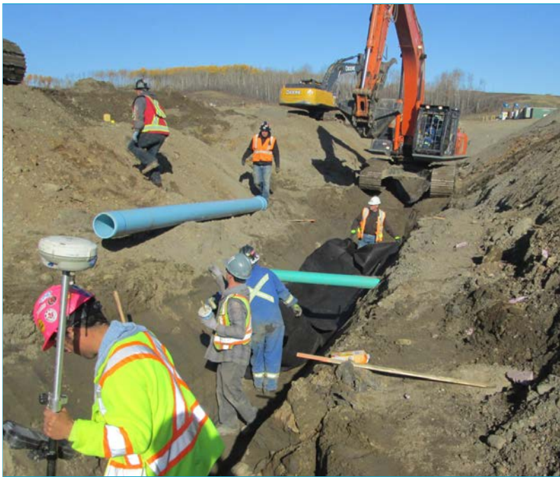
Workers install a water line for the worker lodge.
