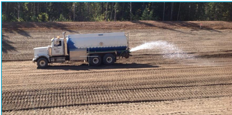
Dust mitigation at the Site C dam site.
