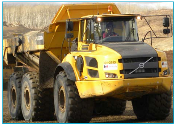
Truck on the north bank of the Site C dam site hauling materials.
