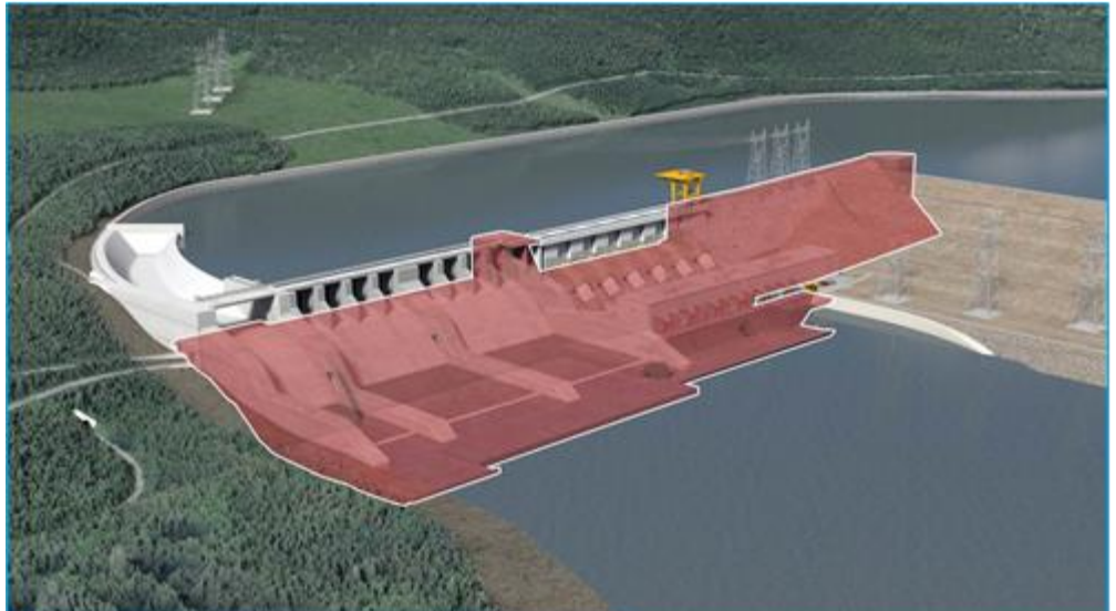
The south valley wall under the dam, the generating station and ancillary structures, and the spillways will be reinforced with a long concrete buttress to improve foundation stability and seismic protection.
