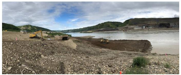
A haul truck (centre) transports material that will be placed on the upstream cofferdam base and spread out by the bulldozer (right). See more project photos in the <u>image gallery</u>.
