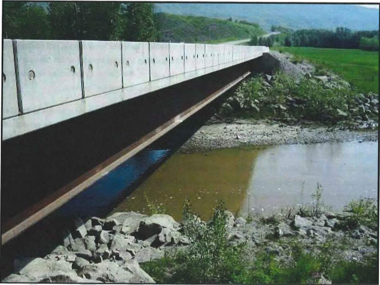
Photograph 2.6.2: Existing Cache Creek Bridge (Credit: AMEC)
