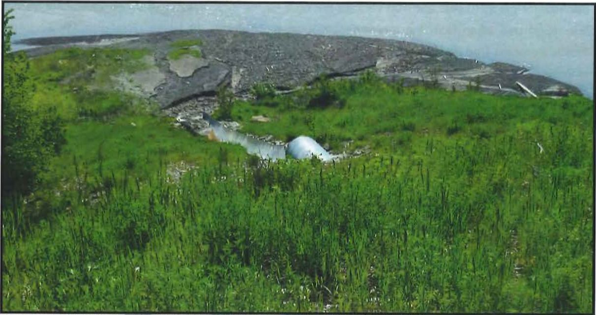
Photograph 2.1.1: Example of pipe outfall in Lynx Creek (Credit: Binnie)
